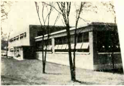
▲ Plant of Westchester manufacturing subsidiary, Pleasantville Instrument Corporation; additions are under construction.
